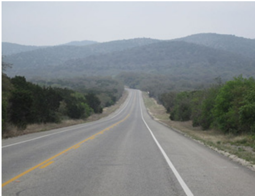
Source: US Hwy. 83 in Uvalde County, TX IMG 1874, Billy Hathorn, Wikimedia
